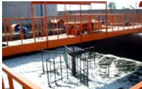
Sprinkling of EM in the equalization tank
