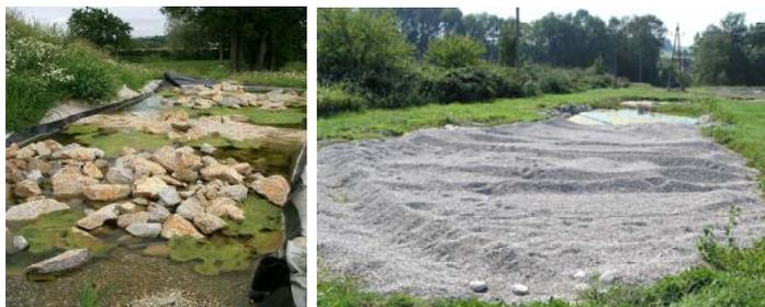
Figure 3. Cascade of retention ponds. The right picture shows the gravel-sand bedding.
